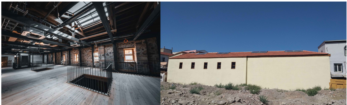
Fig. 2. Photographs from the Current State of the historical akin passage. (left) interior view from the first floor [50] (right) exterior view (source: authors).
